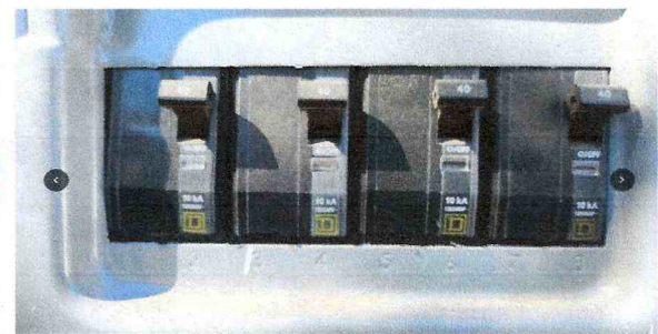
INTERRUPTOR TERMOMAGNETICO 2 X 40 AMP
